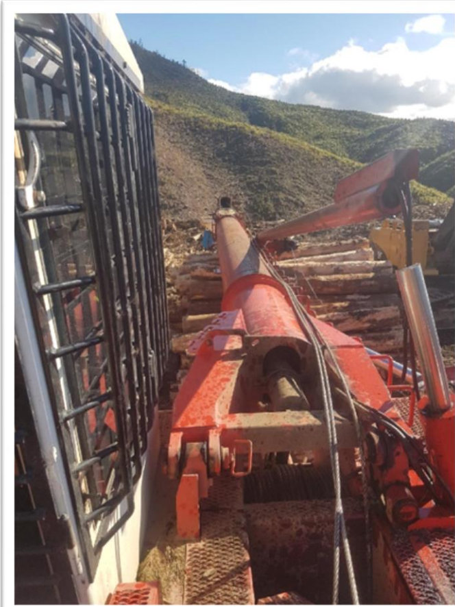
Photo 1: Tower rearward collapse
