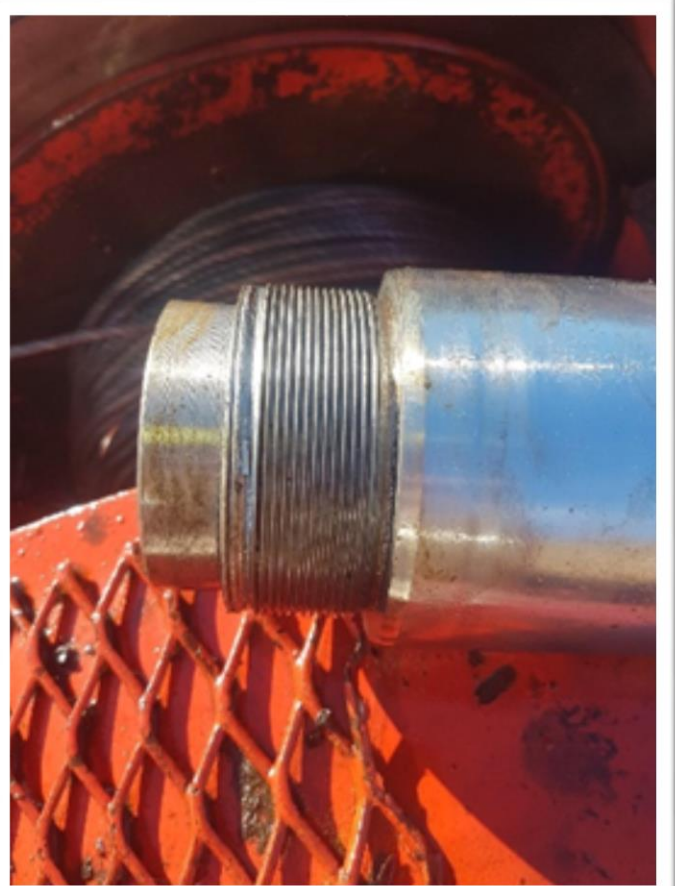
Photo 2: Thread separation on stabiliser ram
